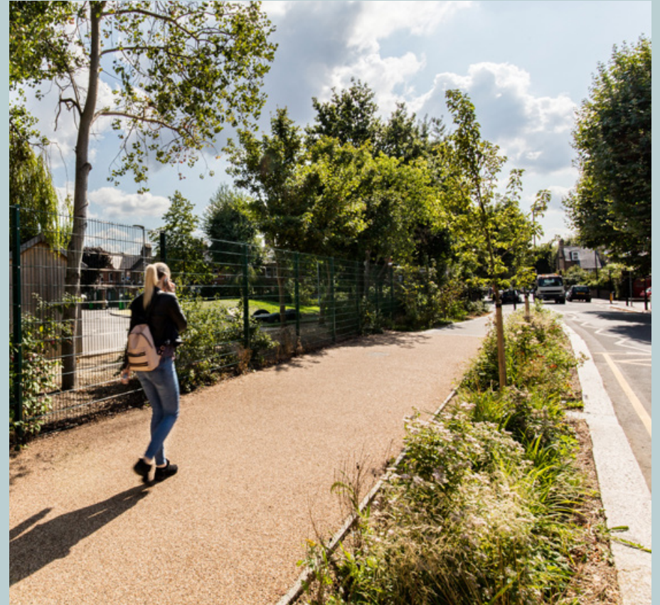
Pretoria Avenue footway widening and rain garden planting. Image photo credit: © Alexander Christie. Scheme design: LBWF Highways in collaboration with what if; projects Ltd.
