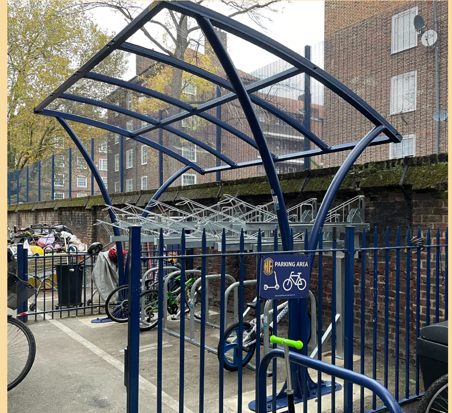
Installed cycle shelter at Henry Fawcett Primary School. © GAP
